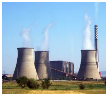
Power Generating Stations
