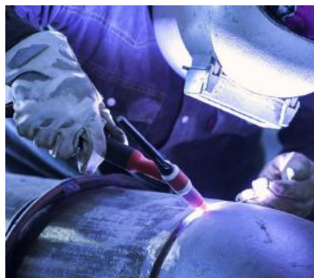
Fabrication & Welding Shops
