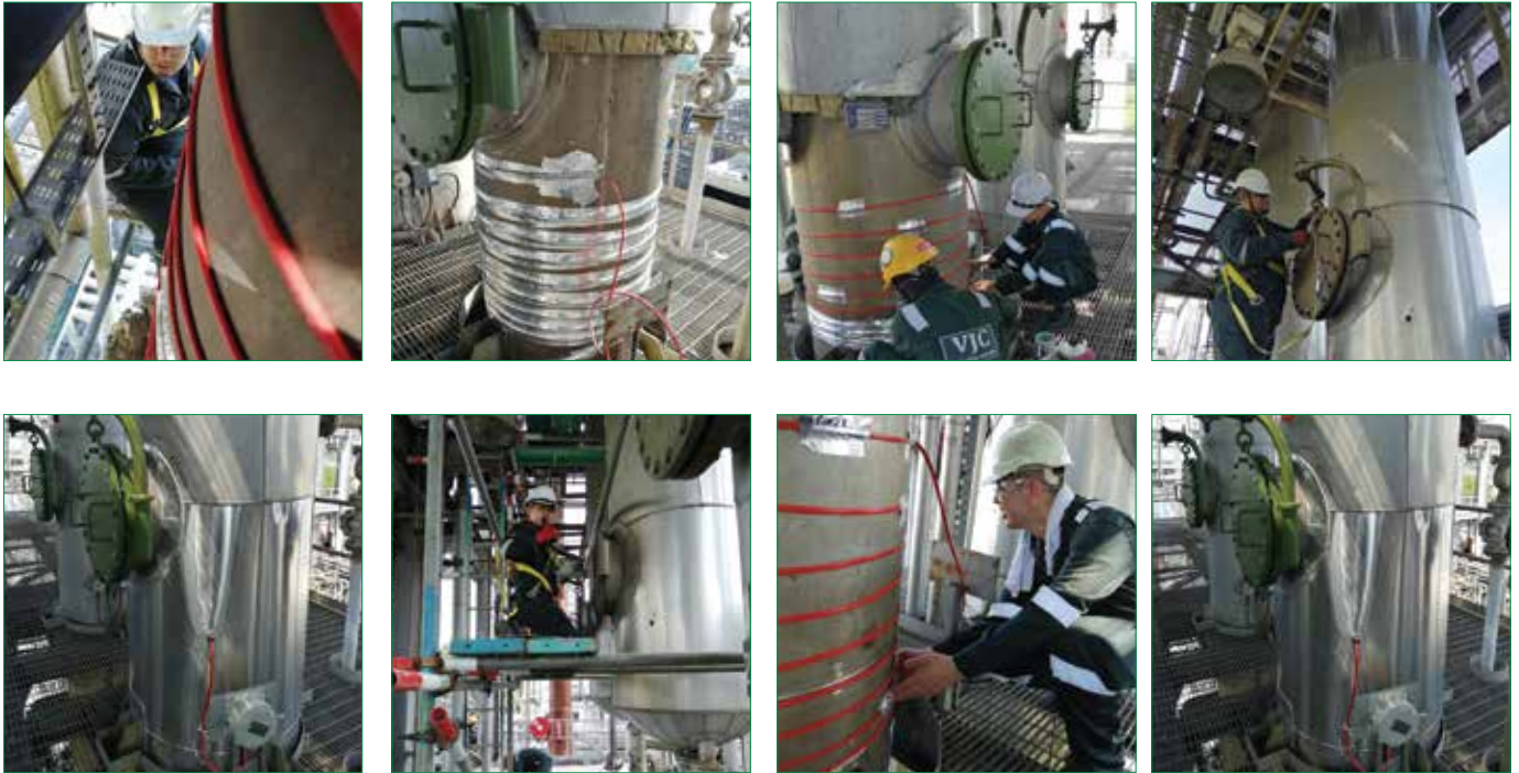
Installing New Heat Tracing Wire And Thermostat Enclosure, Testing & Commissioning
